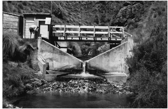
Figure 5.11 A V-notch weir. The water level in the pond behind the weir is recorded continuously.
