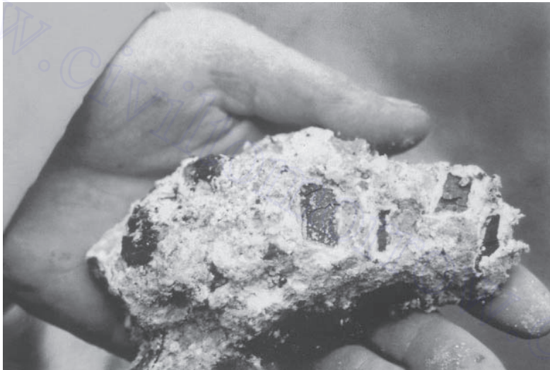
Figure 5.13 A severe example of the thaumasite type of sulphate attack in a hand specimen of concrete.
