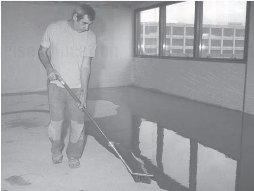
Figure 2.22 Application of floor-levelling compound.
